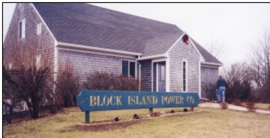
The administrative office of Block Island Power Company.
